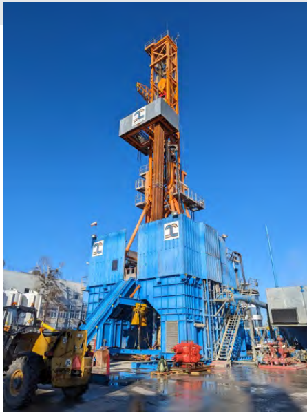
Thermal water approximately 2 km underground is set to largely replace MTU's current gas-based heat supply at the Munich HQ. Credit: MTU
